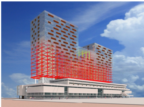
Figure 10. De Karel Doorman in Rotterdam, rendering including structural system (Source: Royal HaskoningDHV)
